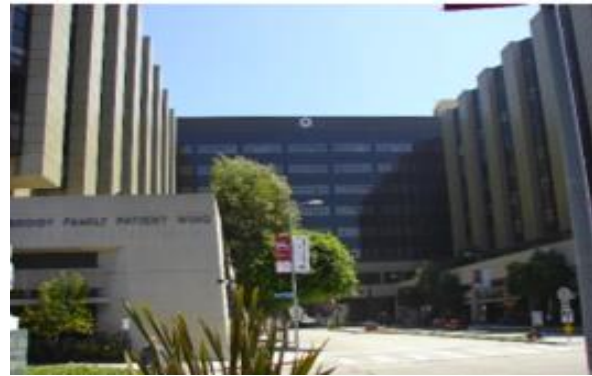
At the Cedars-Sinai hospital campus, alarms help staff protect themselves and patients, and secure hazardous tools and equipment.
